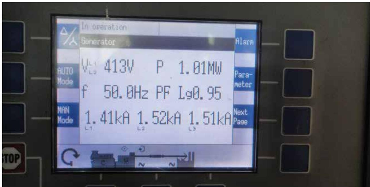
**Picture 7:** A view of control panel readings for power generation values
