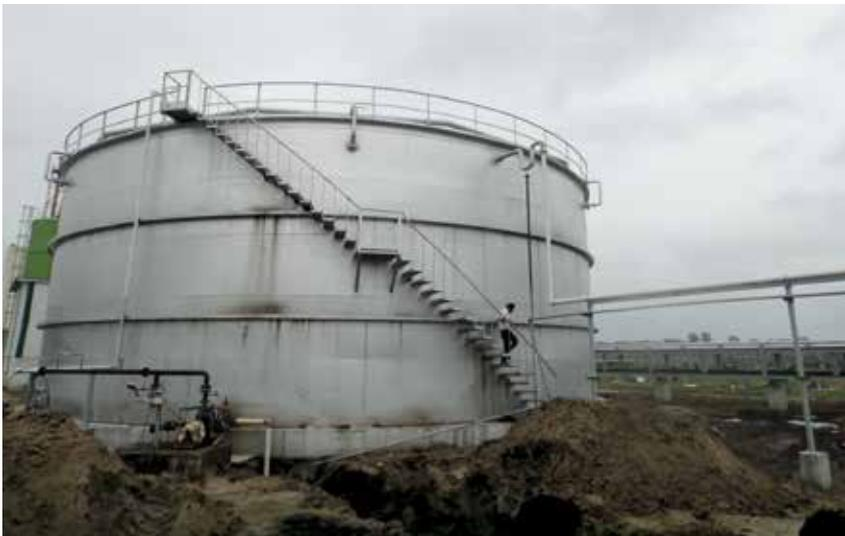
**Picture 4:** A visual of continuously stirred tank reactor digester of 2,000 m<sup>3</sup>
