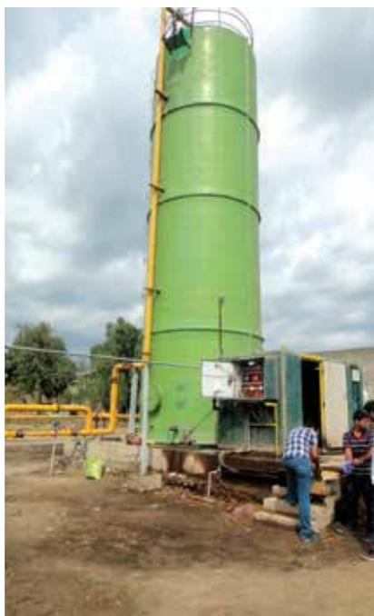
**Picture 5:** A visual of installed hydrogen sulphide biological scrubber
